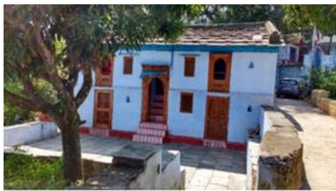
Figure 4. In place of daan (semi-open room on the ground floor) closed rooms are constructed
